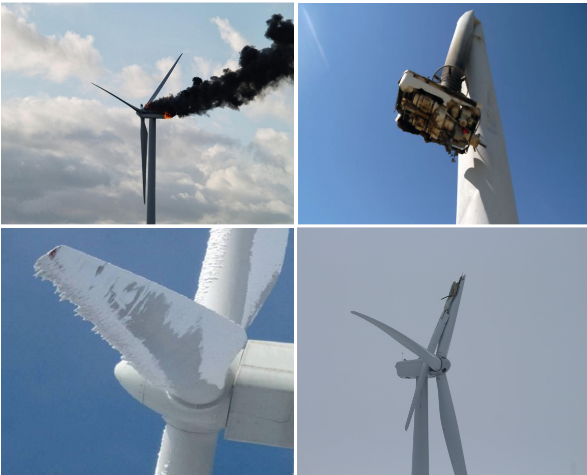
Figure 30. Possible wind turbine accidents (fire: top left; thunder strike and the tower snapping in half: top right; ice on the propeller: bottom left; the propeller snapping: bottom right) (Source: PEI, 2017).
