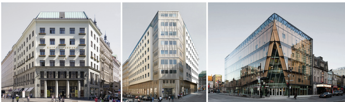
Слика 9. Повлачење угла: 1) Goldman & Salatsch Building - Looshaus, Vienna (Adolf Loos, 1912), 2) Verbund Headquarters, Wien (Solid Architecture, 2010), 3) Quartier Des Spectacles, Montreal (Aedifica, 2012) (Извор: www.archdaily.com) / Figure 9. Corner withdrawal: 1) Goldman & Salatsch Building - Looshaus, Vienna (Adolf Loos, 1912), 2) Verbund Headquarters, Vienna (Solid Architecture, 2010), 3) Quartier Des Spectacles, Montreal (Aedifica, 2012) (Source: www.archdaily.com)
