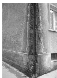
Figure 8. Consequences of the groundwater level rise in the New Belgrade block 7/3
