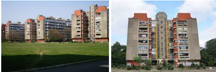
Figure 1: View of the Block 29 residential complex
